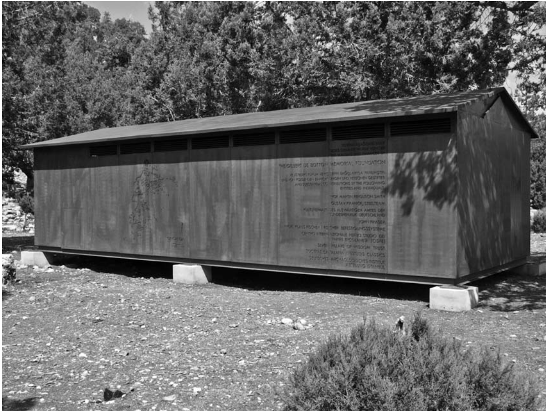
Fig. 1. The storehouse, view from SW
